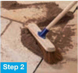
Step 2 With a soft brush/broom, push Pointfix mixture into the gaps.
