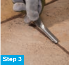
Step 3 Compact firmly into joints using a jointing tool.
